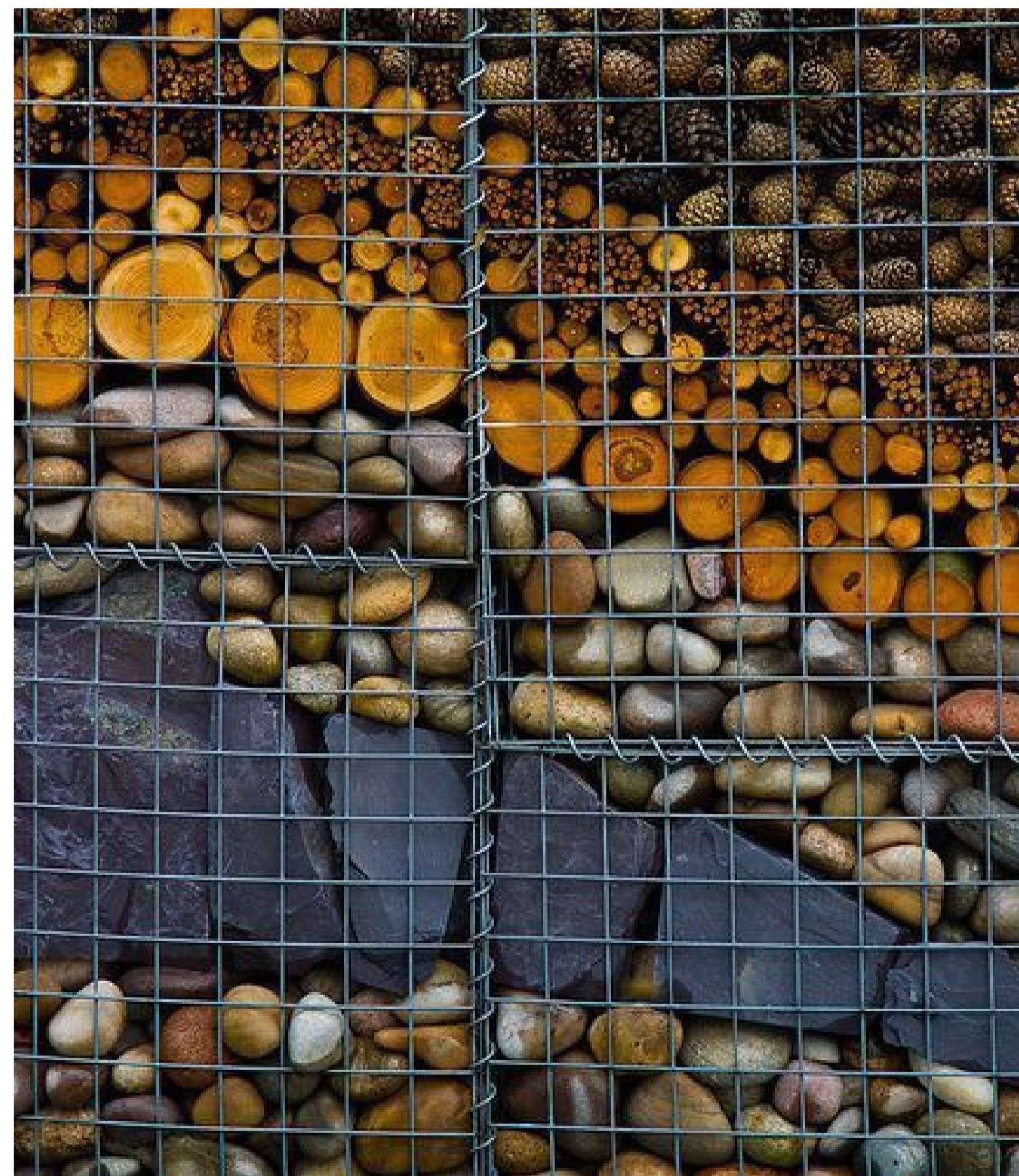
GABION BASKETS 450X450MM FILLED WITH A MIX OF MATERIALS SUCH AS BOULDERS, BRICKS, TIMBER AND PLANTING TO CREATE HABITAT WALLS FOR WILDLIFE
