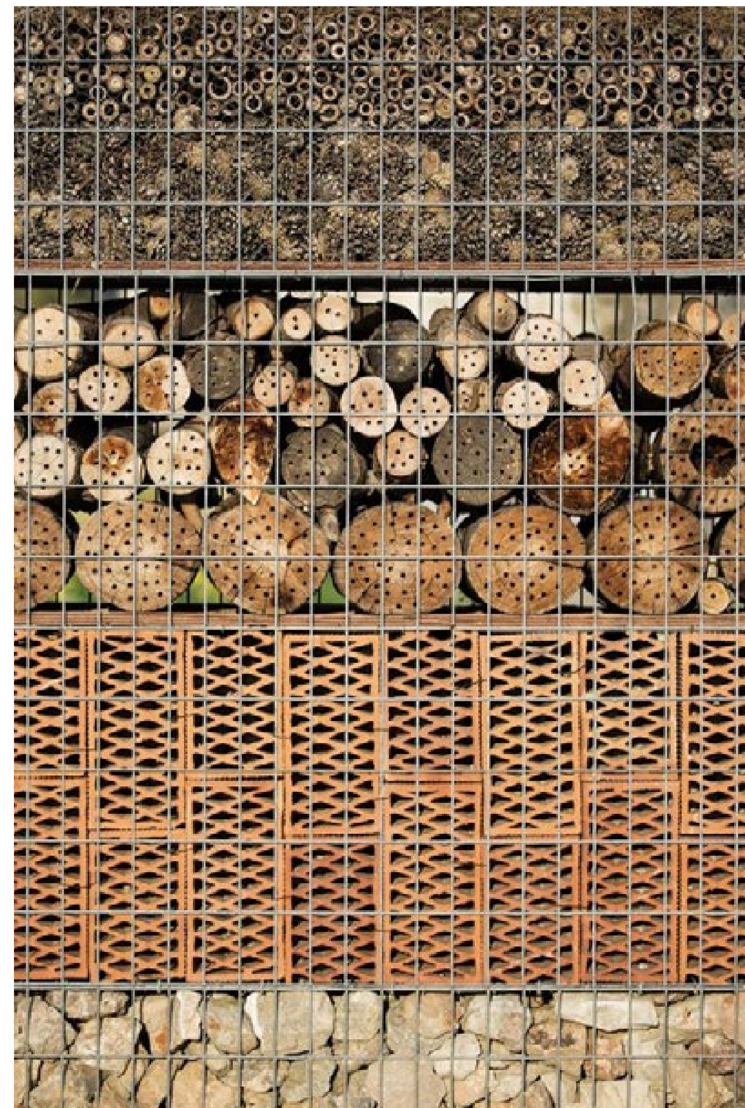
GABION BASKETS 450X450MM FILLED WITH A MIX OF MATERIALS SUCH AS BOULDERS, BRICKS, TIMBER AND PLANTING TO CREATE HABITAT WALLS FOR WILDLIFE
